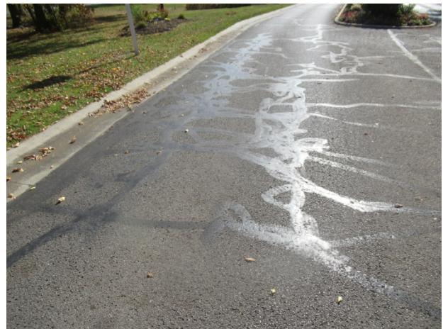
Repaired cracks and settlement near the entrance monument island
