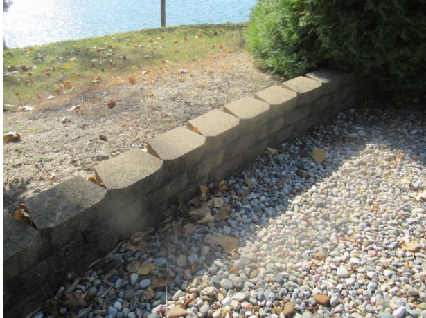
Interlocking block masonry retaining wall at North Moon Lake Drive
