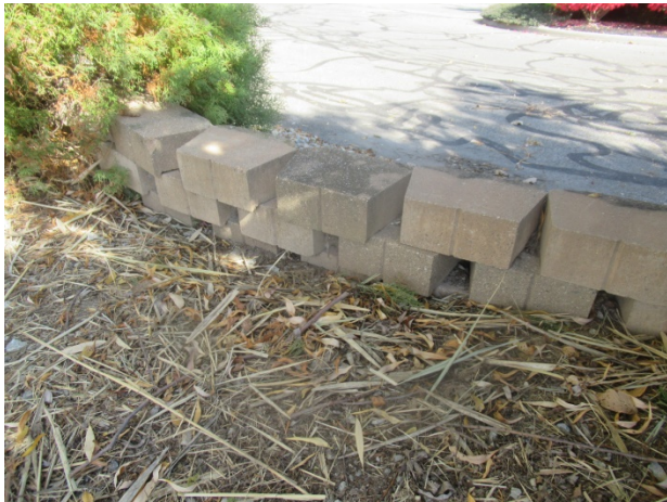
Back side of the wall
