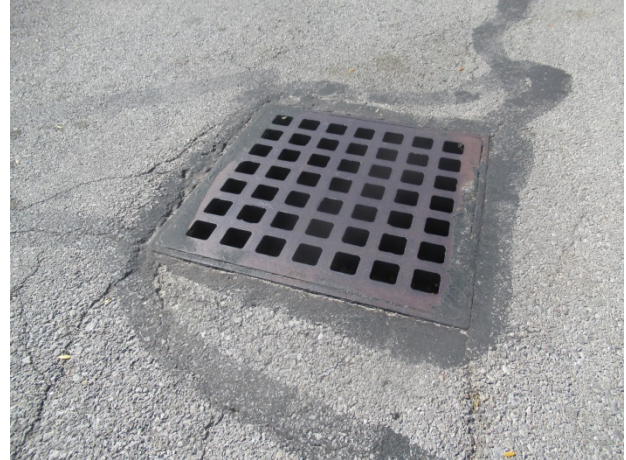
Catch basin at the center of the pavement
