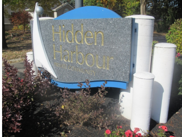
Stone entrance monument sign and concrete pillars
