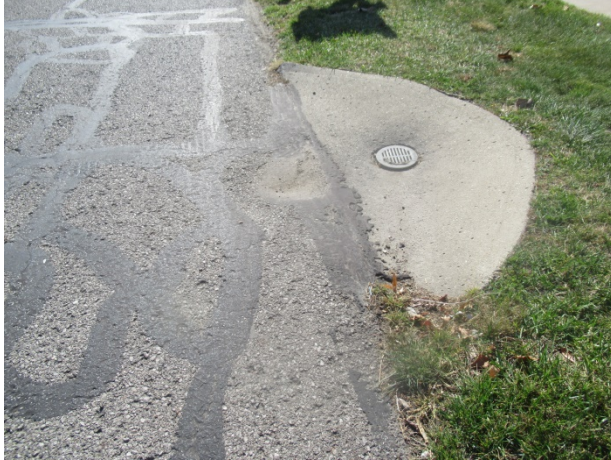
Catch basin at the side of the pavement
