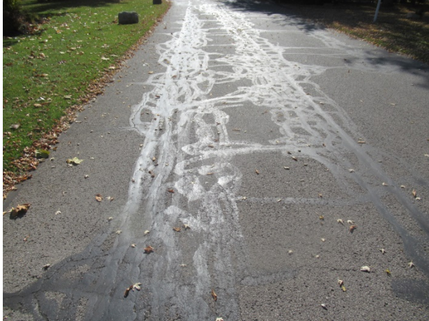
Extensive crack repairs at shared portion
