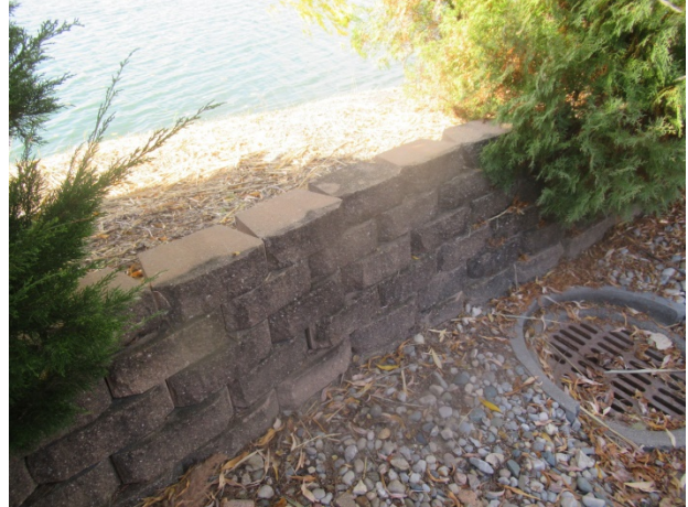
Retaining wall blocks in good condition
