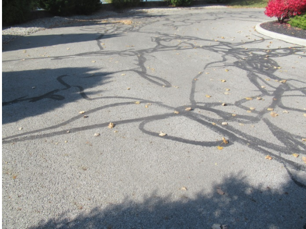
Extensive crack repairs throughout North Moon Lake Drive cul-de-sac
